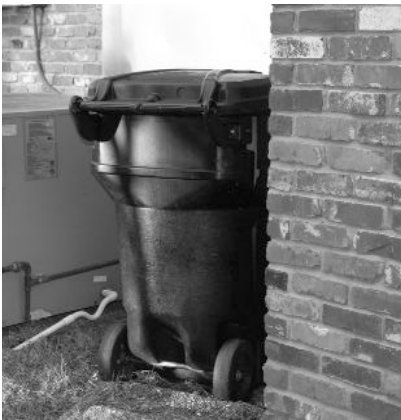
A trash container in need of a screen
